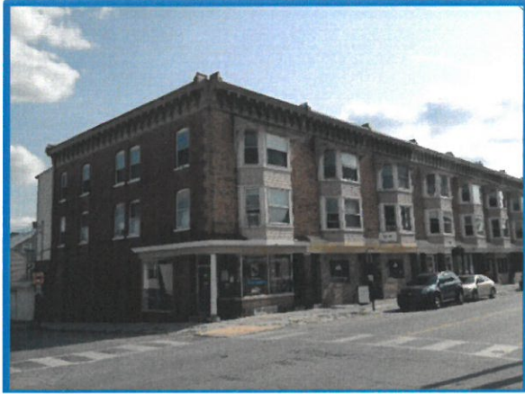
Figure 2-5 (left) and 2-6 (right): Front and rear views of a mixed-use occupancy in downtown Parkesburg often referred to as a “taxpayer” which has commercial and business uses on the first floor and apartments on the upper two floors, creating a significant life hazard and fire control problem.
