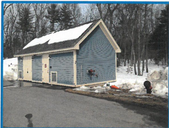
Figures 2-20 and 2-21: Pump house and fire department connections to access water in below ground cistern stored for firefighting use in a planned subdivision in Berlin, MA. The Keystone Valley Fire Department should consider encouraging their member townships to adopt a proactive fire and life safety regulation requiring these in any planned subdivision of three or more homes, and for any home that exceeds a certain designated square footage.
