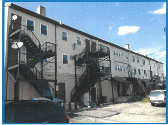
Figure 2-5 (left) and 2-6 (right): Front and rear views of a mixed-use occupancy in downtown Parkesburg often referred to as a “taxpayer” which has commercial and business uses on the first floor and apartments on the upper two floors, creating a significant life hazard and fire control problem.
