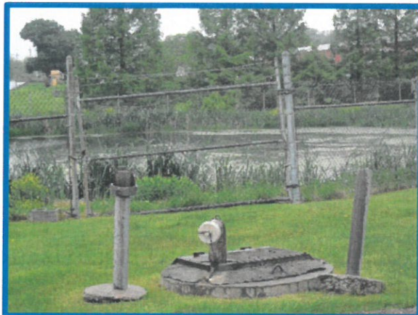
Figure 2-18 (left): Dry hydrant/standpipe on Route 30 designed to make drafting water from the pond in the background quicker and easier for fire personnel.
